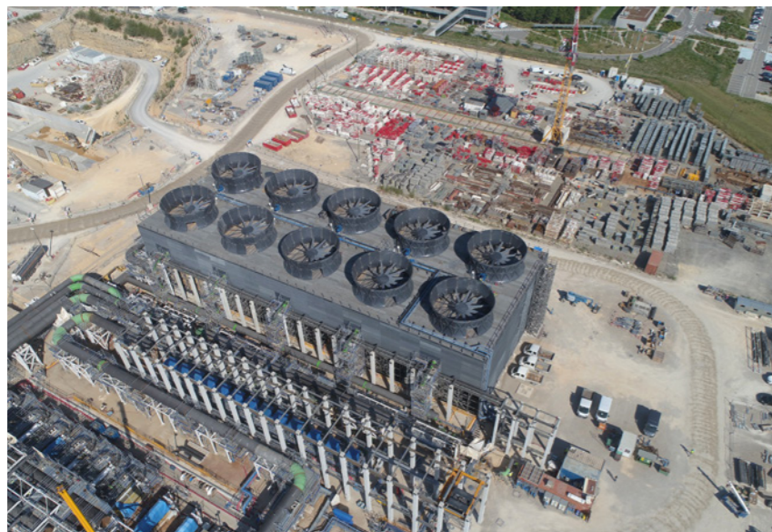
Ten fans installed at the top of the building, one for each cooling tower. Cooling basins passed fill tests.
