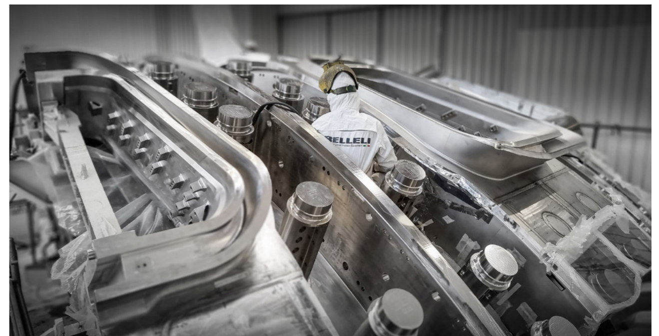
Working on the final assembly of segment 2-sector 3 of Europe's contribution to the ITER Vacuum Vessel. Works performed at Belleli, Mantova, Italy © Belleli
