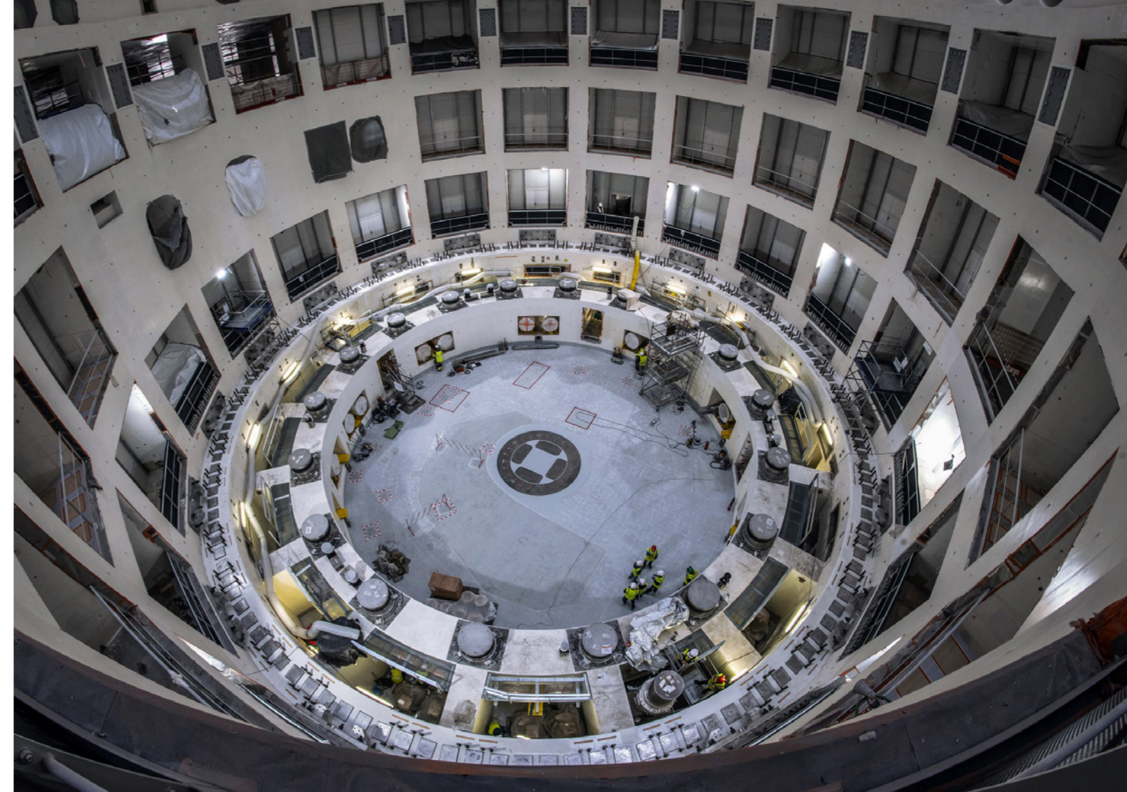
Tokamak pit unveiled ready to receive the Cryostat lower base. The 18 cylindrical support bearings are visible. ITER site, Cadarache, France, May 2020 © ITER Organization
