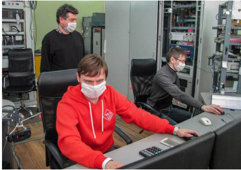
Factory acceptance tests completed for fourth gyrotron set.
