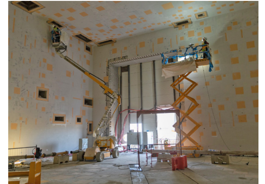
A constellation of embedded plates. One can guess at the number of components that will be installed in this large room by the number of anchor plates on the walls, ceiling and floor. © Les Nouveaux Médias/SNC ENGAGE
