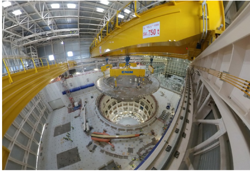
First major machine component—the cryostat base—lifted by overhead crane and lowered into the Tokamak assembly pit.
