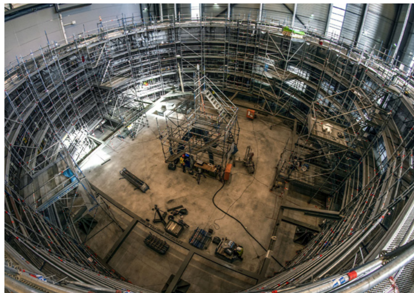
430-tonne upper cylinder of Cryostat completed.
