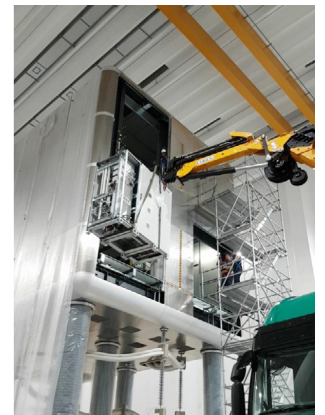
Inserting part of MITICA's Ion Source and Extraction Power Supplies (ISEPS) in the High Voltage Deck © F4E
