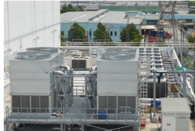
Aerial view of the cooling towers and air coolers, part of the European contribution to the ITER Neutral Beam Test Facility, Padua, Italy © F4E
