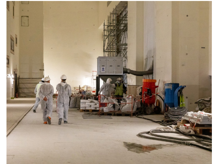
Painting works advancing in the Tokamak complex. An estimated 150 tonnes of resin, primer and paint are required. ITER site, Cadarache, France, December 2020 © Les Nouveaux Médias/SNC Engage
