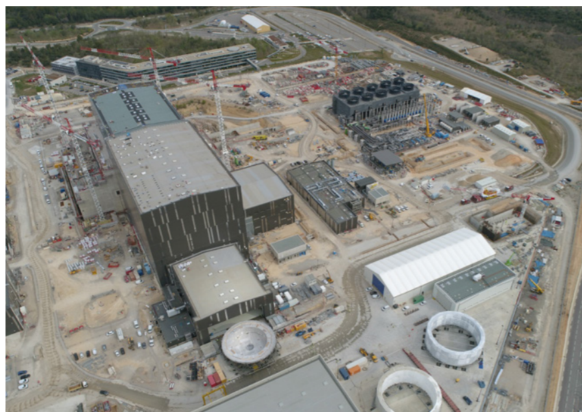
Fusion for Energy officially handed over the ITER Assembly building to ITER Organization. The building's extensive HVAC system is ready to maintain the specific temperature and humidity levels required during machine assembly.
