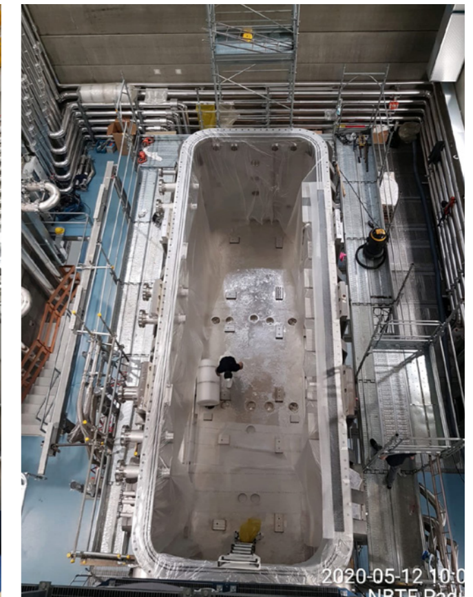
Top down view of the MITICA Vacuum Vessel during the preparatory works before welding operations begin inside the vessel, ITER Neutral Beam Test Facility, Consorzio RFX, Padua, Italy © F4E
