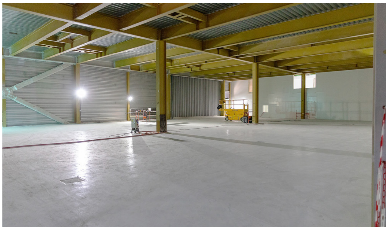
The structure of the three-floor Radio Frequency building is in place to welcome the first equipment that started arriving in summer. The ground floor (pictured) will house 12 power supplies for 24 gyrotrons (external heating devices). © Les Nouveaux Médias/SNC ENGAGE.
