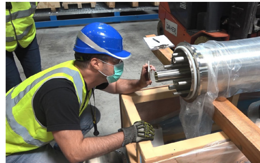
First part of the gas injection system -18 crates of spools—delivered. They will be part of a series of pipes that transports all gases into the Tokamak Building from the tritium plant.
