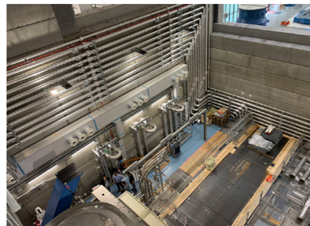
Top down view of the MITICA cooling plant system in the pit of the experiment, ITER Neutral Beam Test Facility, Consorzio RFX, Padua, Italy © F4E
