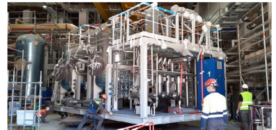
Helium dryer weighing nearly 50 tonnes being rotated into its final position inside the cryoplant buildings. Cadarache, June 2020. © F4E
