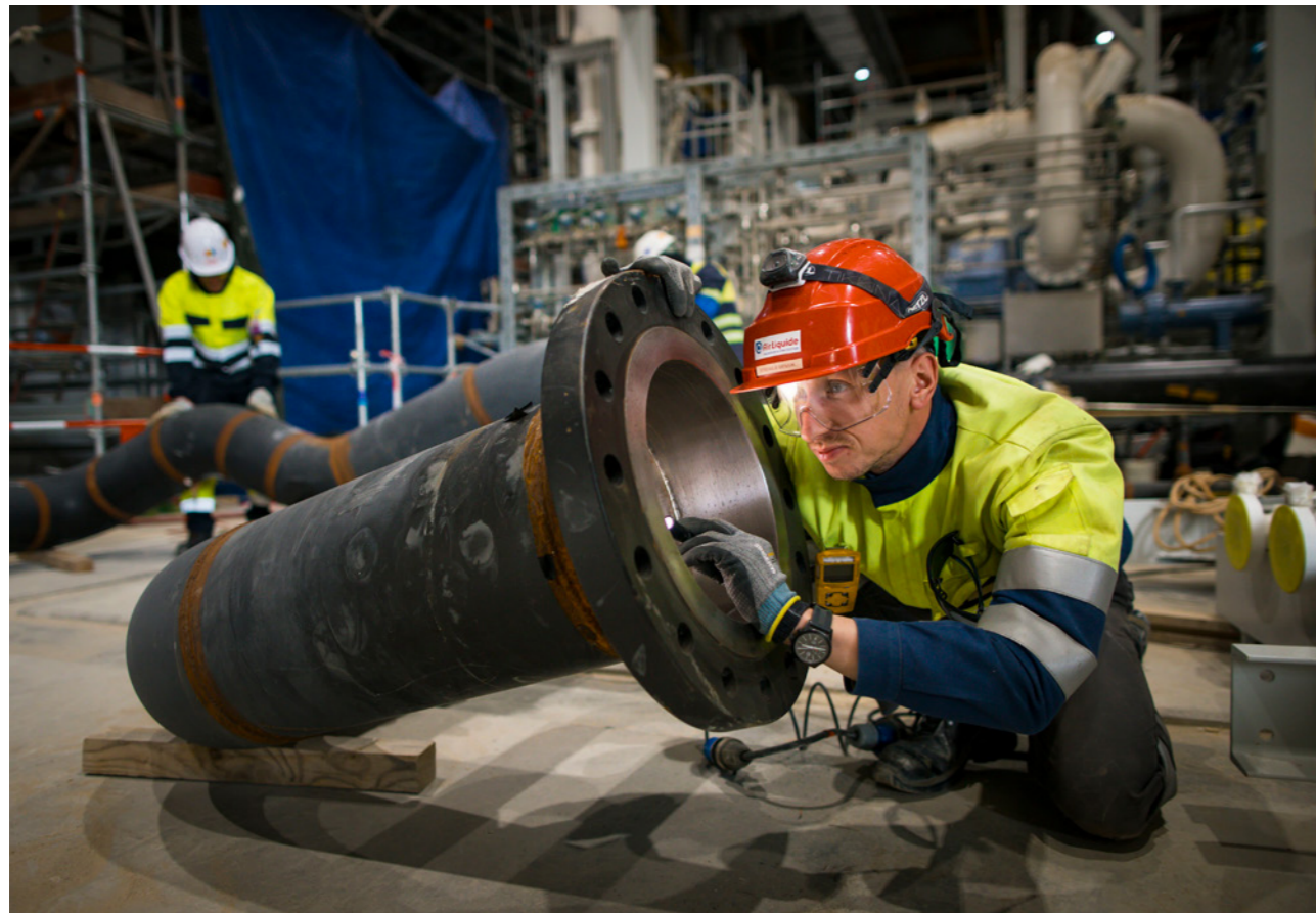
Mykhailo Geniuk (Air Liquide Mechanical Supervisor) inspecting a pipe prior to installation, ITER Cryoplant. Works financed by F4E. Cadarache, November 2019. © F4E
