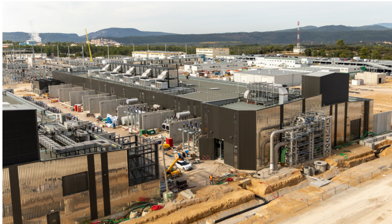
More equipment installed inside and outside of the Magnet Power Conversion buildings to provide DC voltages to the magnets © Les Nouveaux Médias/SNC ENGAGE
