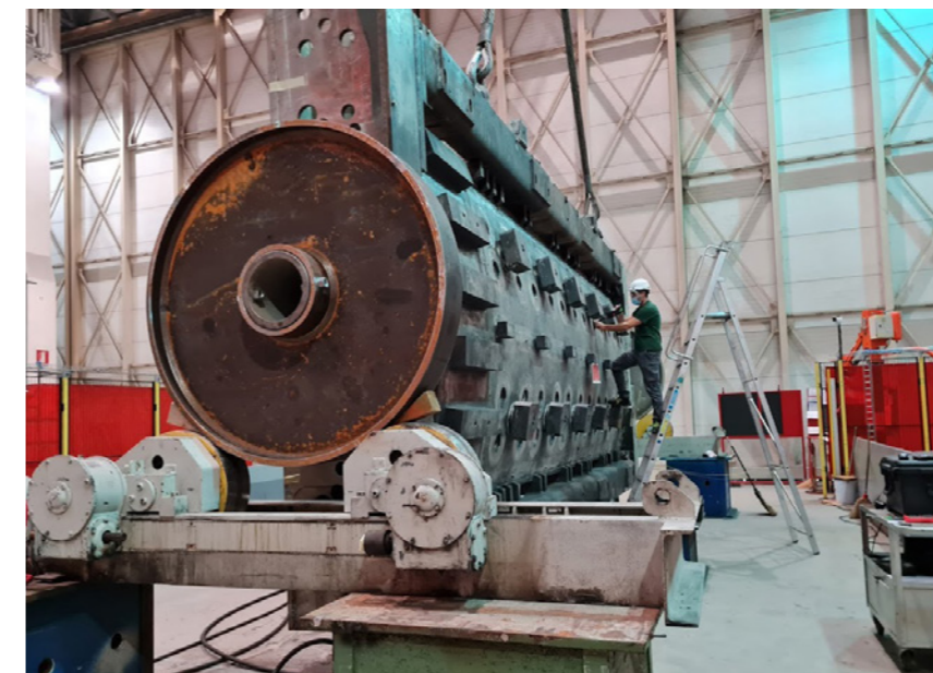
Machining of ITER Vacuum Vessel sector 5, segment 1, Mangiarotti, Monfalcone, Italy © Mangiarotti
