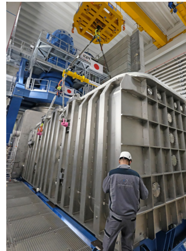
Technician conducting final checks on MITICA Vacuum Vessel prior to hand over, ITER Neutral Beam Test Facility, Consorzio RFX, Padua, Italy, May 2020 © F4E
