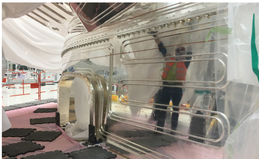
Thermal Shields unwrapped in ITER Assembly Hall
