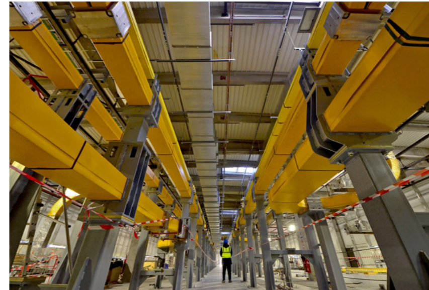
Five kilometres of actively cooled aluminium busbars, procured by Russia, installed in the Magnets Power Conversion buildings.
