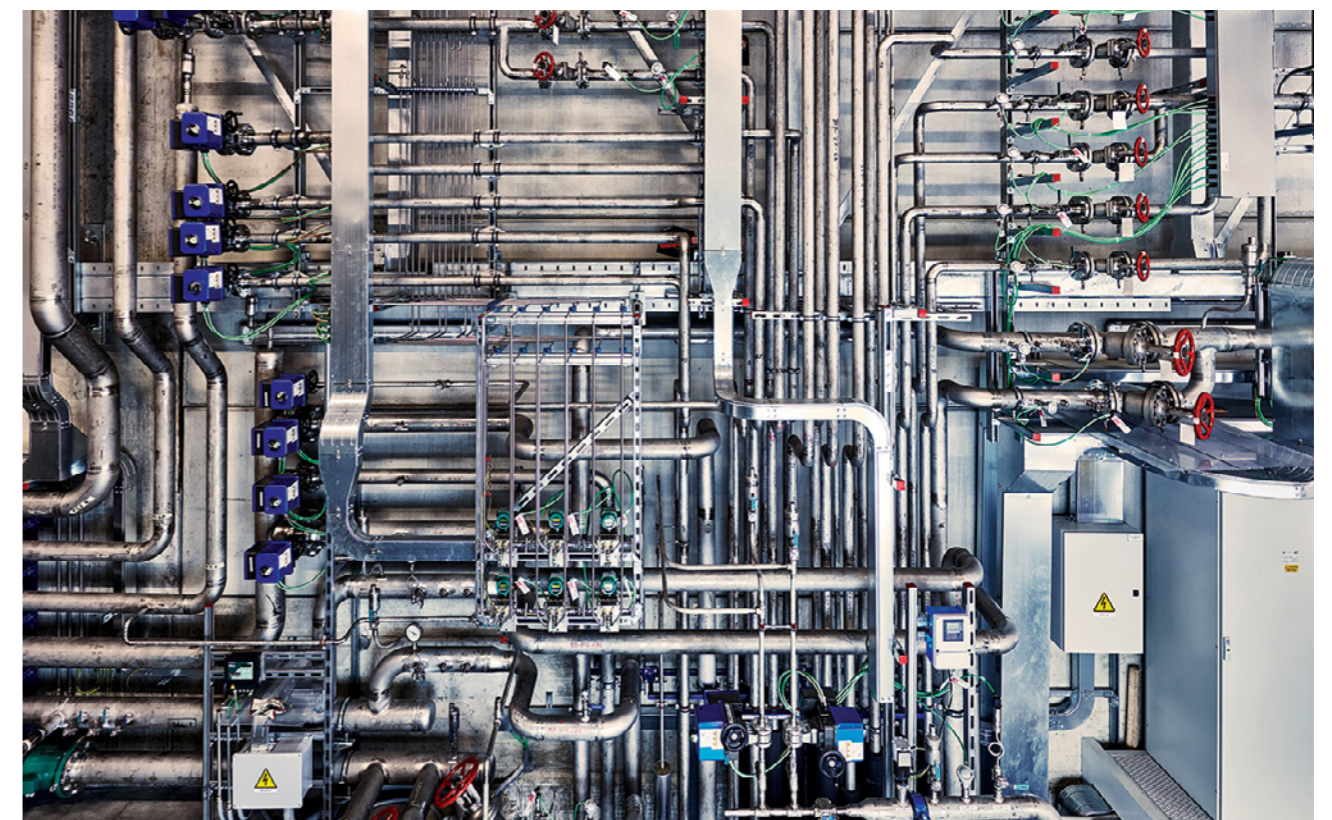
SPIDER Cooling plant, part of the European contribution to the ITER Neutral Beam Test Facility, Consorzio RFX, Padua, Italy Copyright: Enrico Sacchetti
