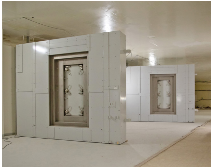
Port cells connect the bioshield to the outlying galleries. For their installation, it was decided to use reinforcement and concreting of the frames, ITER site, October 2020 © ITER Organization
