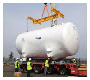
Delivery at ITER site of a 100 m<sup>3</sup> tank
