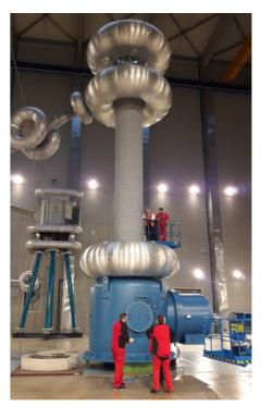
The installation of the High Voltage Deck inside the MITICA High Voltage hall, October 2017. ©
