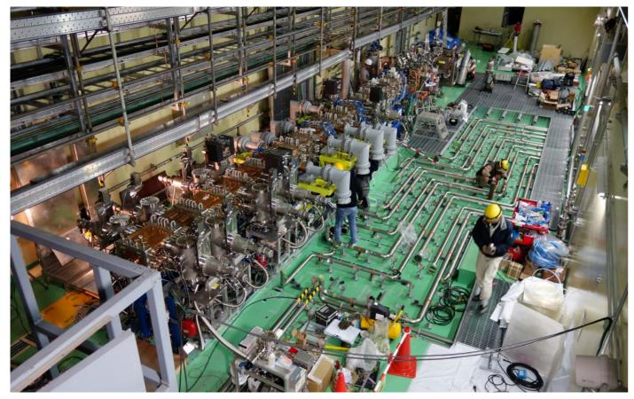
Top view into the LIPAc accelerator vault during the installation of the cooling loops for the "Badiofrequency Quadrupole". Rokkasho, Japan
