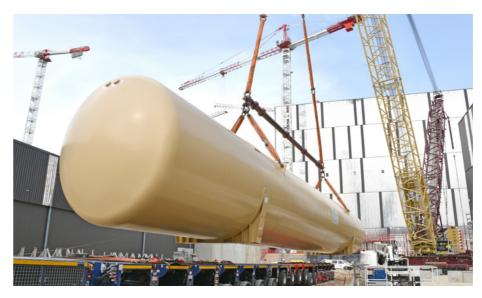
Lifting one of the two quench tanks financed by F4E and produced by Chart Ferox. ITER Cryoplant, April 2018.
