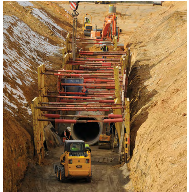
Overflow network - pipes' backfilling
