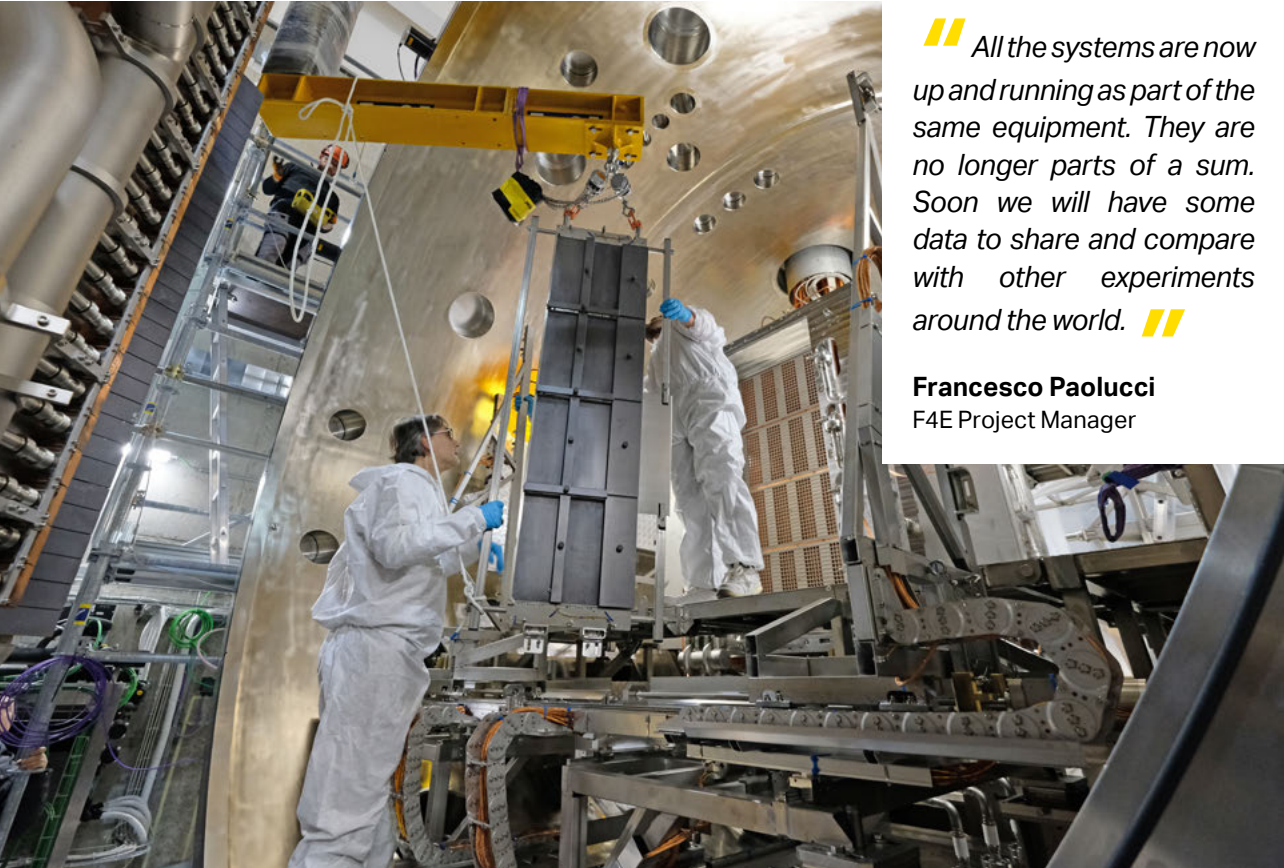
Members of Consorzio RFX installing diagnostics equipment, the STRIKE calorimeter, in SPIDER so as to monitor the operation of the beam source, March 2019, Padua, ITER Neutral Beam Test Facility.
