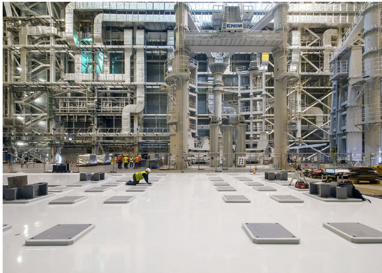
Inside the Assembly Hall, piping and HVAC testing are performed whilst other contractors are coating its 6 500 m 2 floor with epoxy resin, Cadarache, France, October 2019 © ITER Organization
