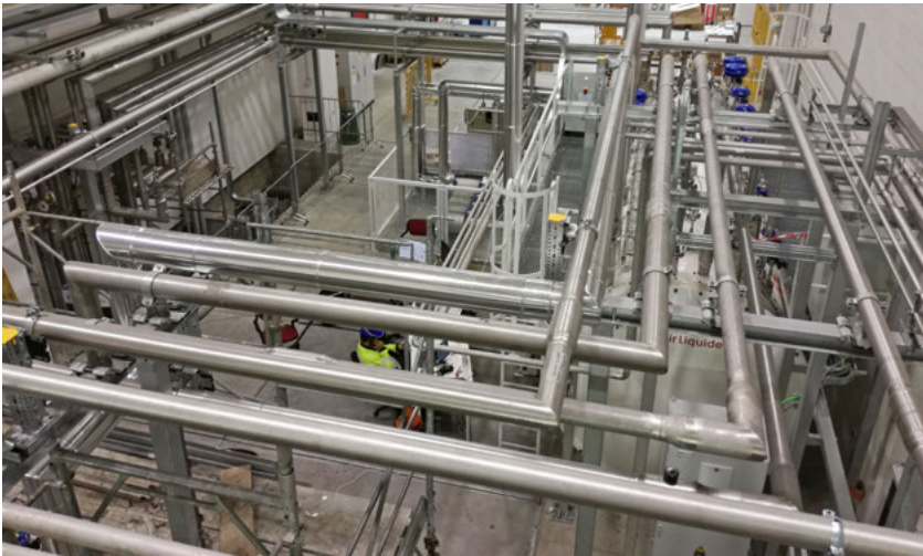
Cryolines connecting the main cold box with the auxiliary cold box, ITER Neutral Beam Test Facility, MITICA, Padua, Italy
