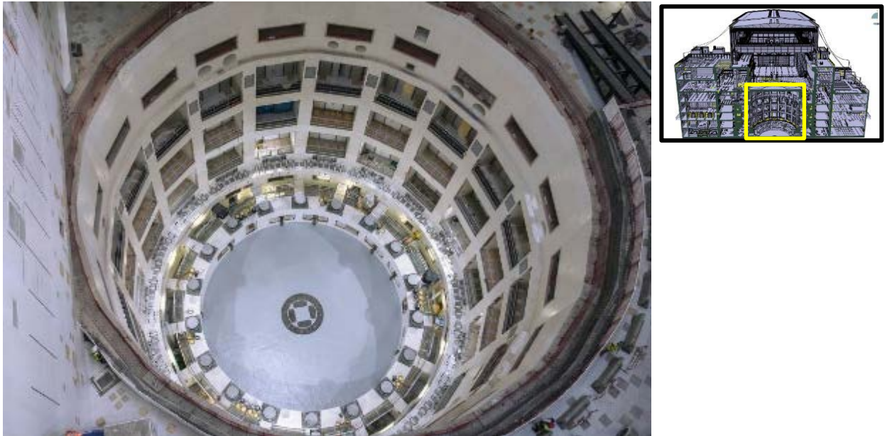
Figure 2: Bioshield, Concrete Crown and Pit Completed and handed over to IO ready for Cryostat Base lifting
