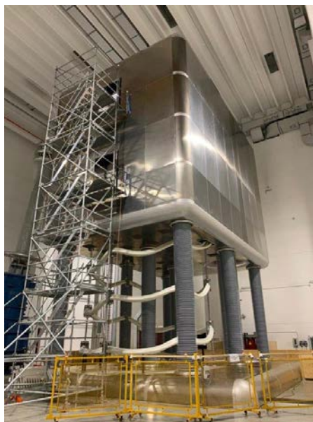
Figure 36: MITICA ISEPS installed inside the HV Deck
