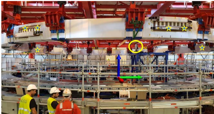
Figure 58: Real Time Positioning of PF2 from Station E to Station F
