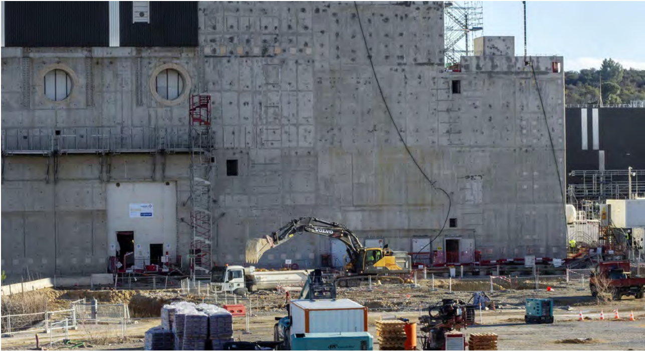
On a level area in front of the Tokamak Complex, excavation works started for a series of buildings that will be dedicated to the power supply of the ITER Neutral Beam heating system, ITER construction site, Cadarache, France, January 2022. © ITER Organization
