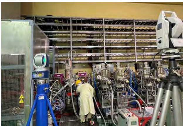
Realignment of a magnet in the Low Energy Beam Transport (LEBT) line. Japan, March 2021. © IFMIF/EVEDA
