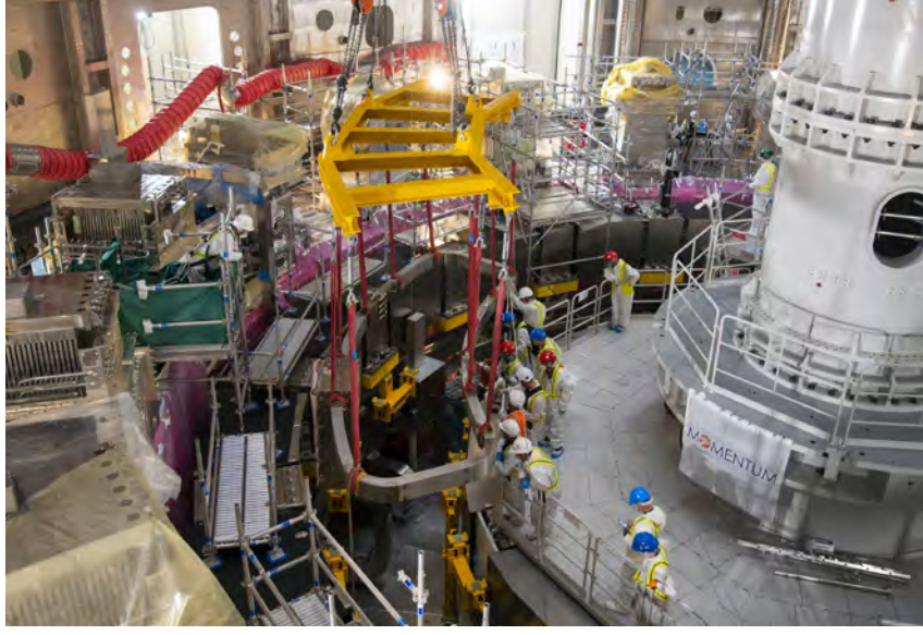
Lowering of correction coil 4 in the Tokamak pit. The space between Poloidal Field coil 5, Poloidal Field coil 6, lower magnet feeders, and staging platforms does not exceed 25 mm. October 2021 © ITER Organization
