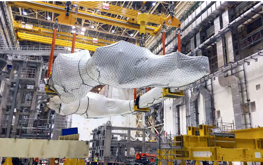
Moving one of Europe's Toroidal Field coils from the transport frame to the storage frame, ITER Assembly Hall, Cadarache, France, July 2021. © ITER Organization
