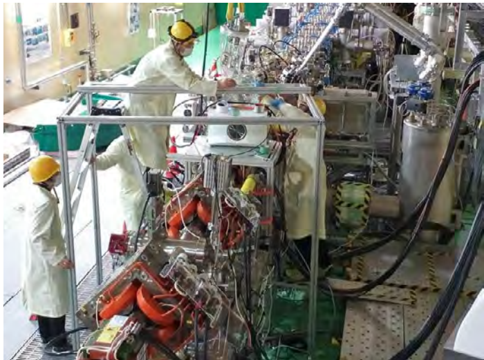
Preparation of sensor installation in the intermediate transport line in place of the cryomodule, Japan, March 2021. © FMIF/EVEDA
