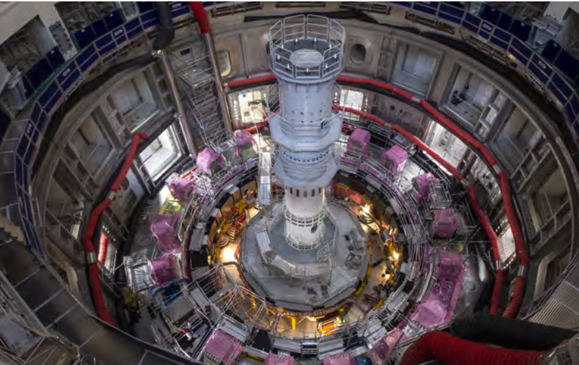
The 30-metre-deep Tokamak pit ready to receive its first 40-degree vacuum vessel section. The central column, equipped with ladders and access ports, will be used to reach different levels of the emerging torus. December 2021 © ITER Organization
