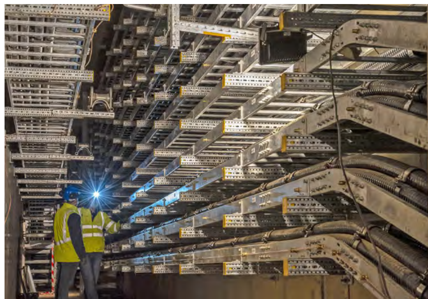
Cables located below the west entrance of the magnet power conversion buildings head in all directions, eventually reaching the four corners of the platform. Procured by China, the cables are delivered in drums and unspooled. February 2021 © ITER Organization
