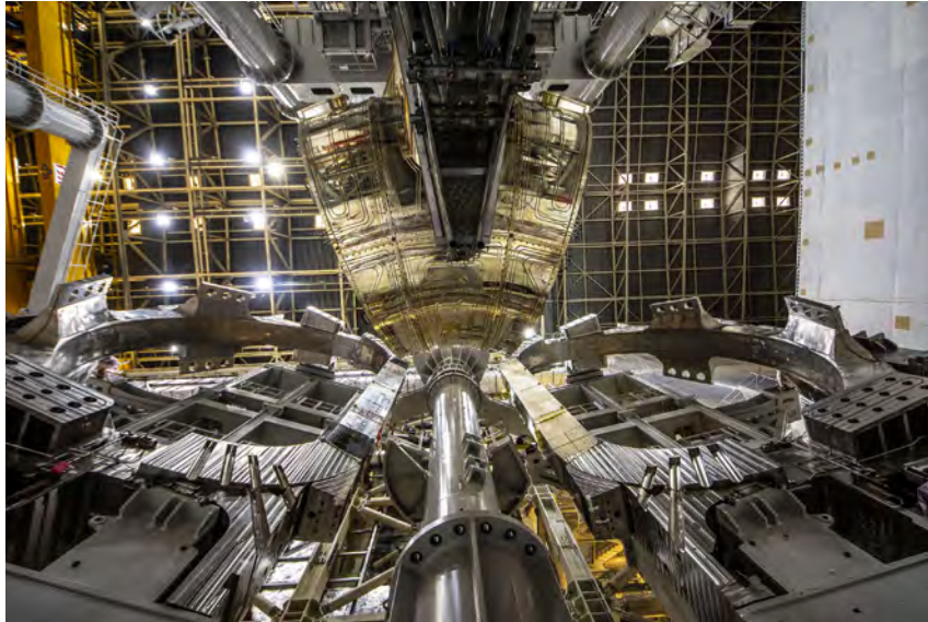
ITER assembly advancing. Tool capable of supporting a vertical vacuum vessel sector (440 tonnes, centre) and two toroidal field coils (2 x 350 tonnes, left and right). September 2021 © ITER Organization
