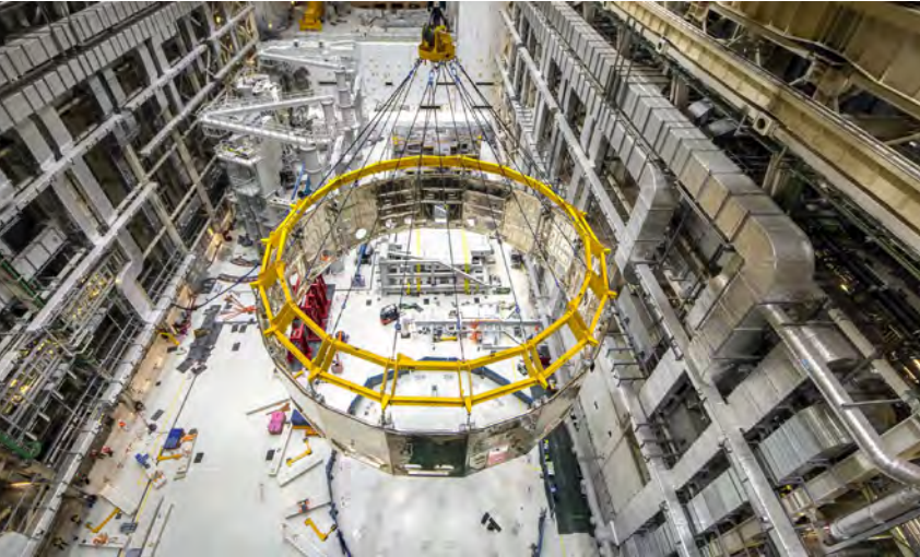
The ITER Assembly and Construction teams successfully lift the cylindrical lower cryostat thermal shield to get inserted in the Tokamak pit, January 2021 © ITER Organization
