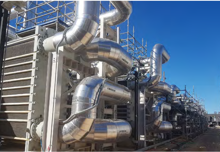
Equipment procured by India has been installed in the 6 000 m 2 Cooling Plant on the northern corner of the ITER site, including heat exchangers as shown in the image. October 2021 © ITER Organization
