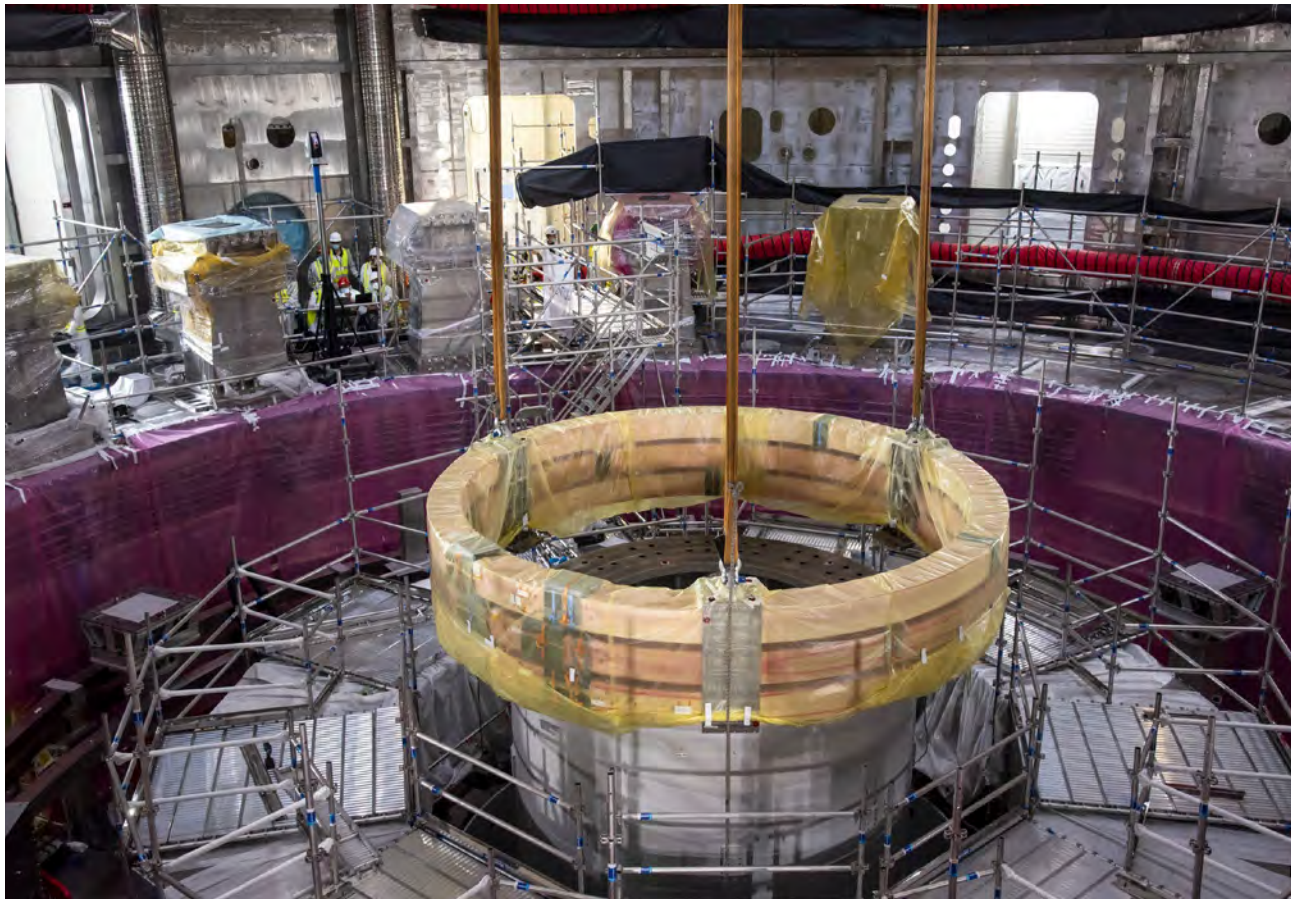
Installation of a set of three spare Pre-Compression Rings in the Tokamak pit, July 2021. Two other sets of three rings will hold tightly the Toroidal Field coils at top and bottom against any expansion forces during operation. © ITER Organization
