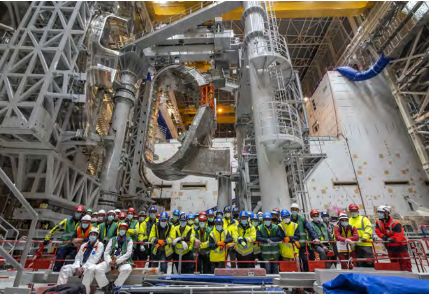
Sector 6 of the ITER Vacuum Vessel, supported by a radial beam above, safely docked in the sector sub-assembly tool, April 2021 © ITER Organization
