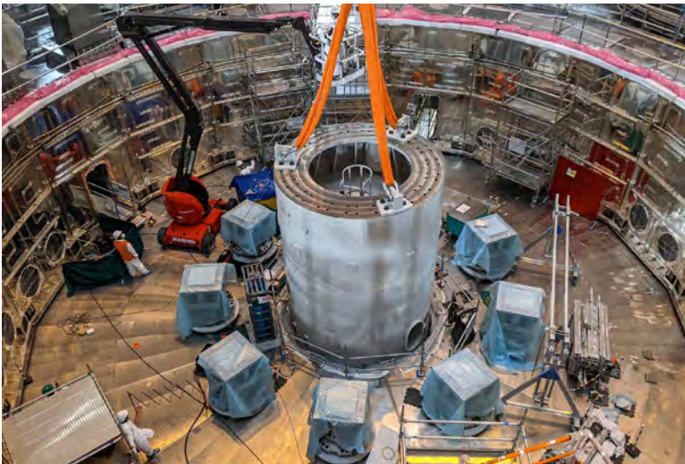
Bottom cylinder of the in-pit assembly tool installed. With a central column and radiating beams braced against the pit walls, the in-pit column tool will support the nine sectors of the vacuum vessel as they are welded together. Cadarache, France, March 2021. © ITER Organization
