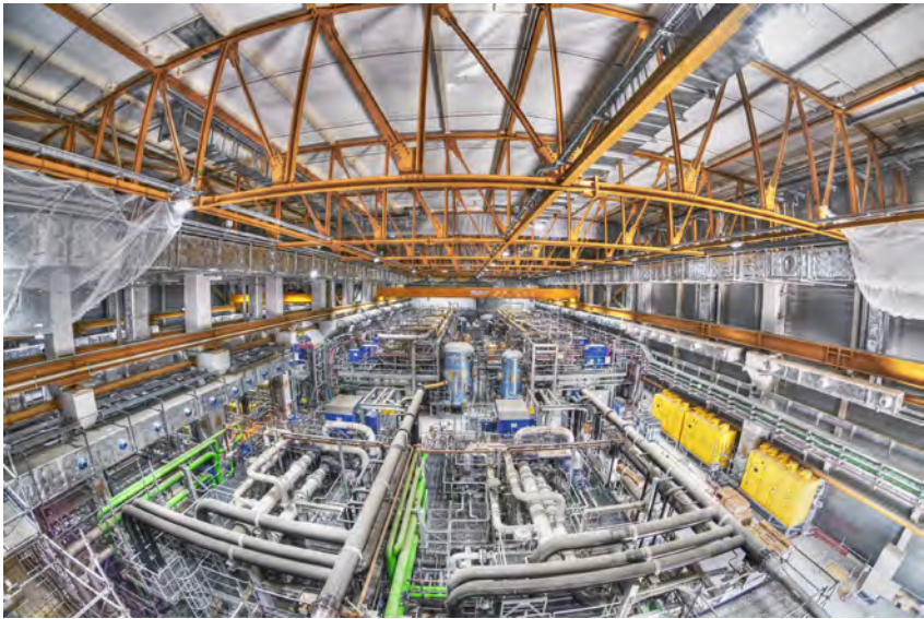
As big as two football pitches, the cryoplant provides cooling fluids for the superconducting magnets, the cryopumps, and thousands of square metres of thermal shielding, Cadarache, March 2021. © Christian Lünig
