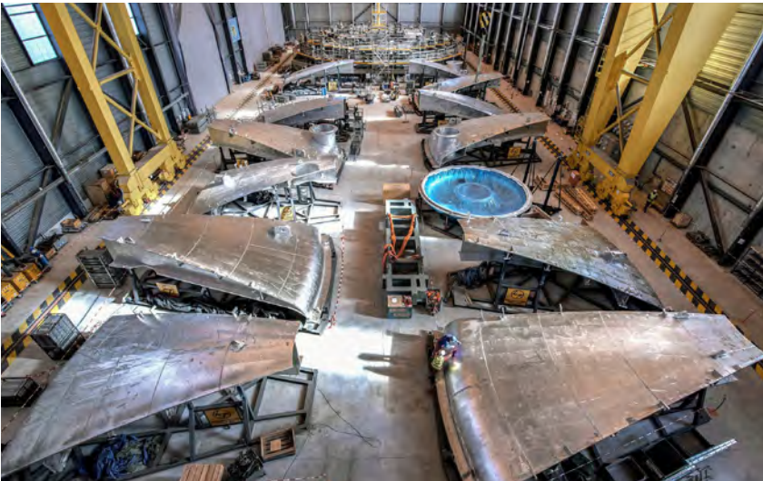
Major elements of the cryostat top lid produced by India, aligned on the floor of the workshop. February 2021 © ITER Organization
