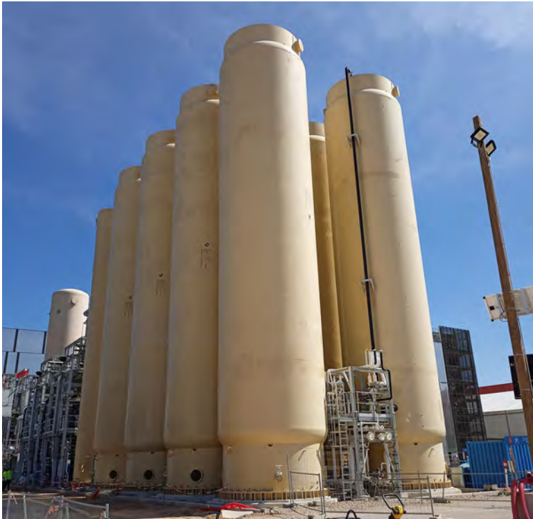
Gaseous helium storages that would be enough to fill 4 million party balloons. Cadarache, September 2021. © F4E
