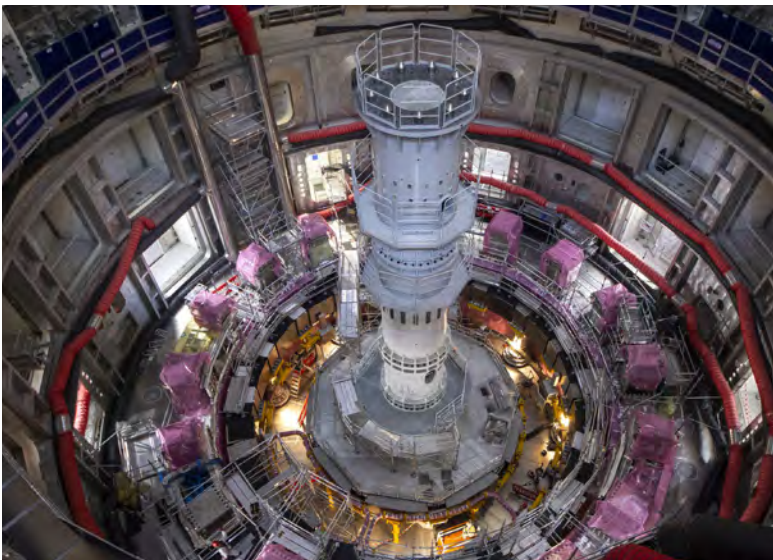
The central column of the in-pit column tool is in place. The nine radial beams will arrive next to support a vacuum vessel sub-assembly. Cadarache, France, December 2021. © ITER Organization
