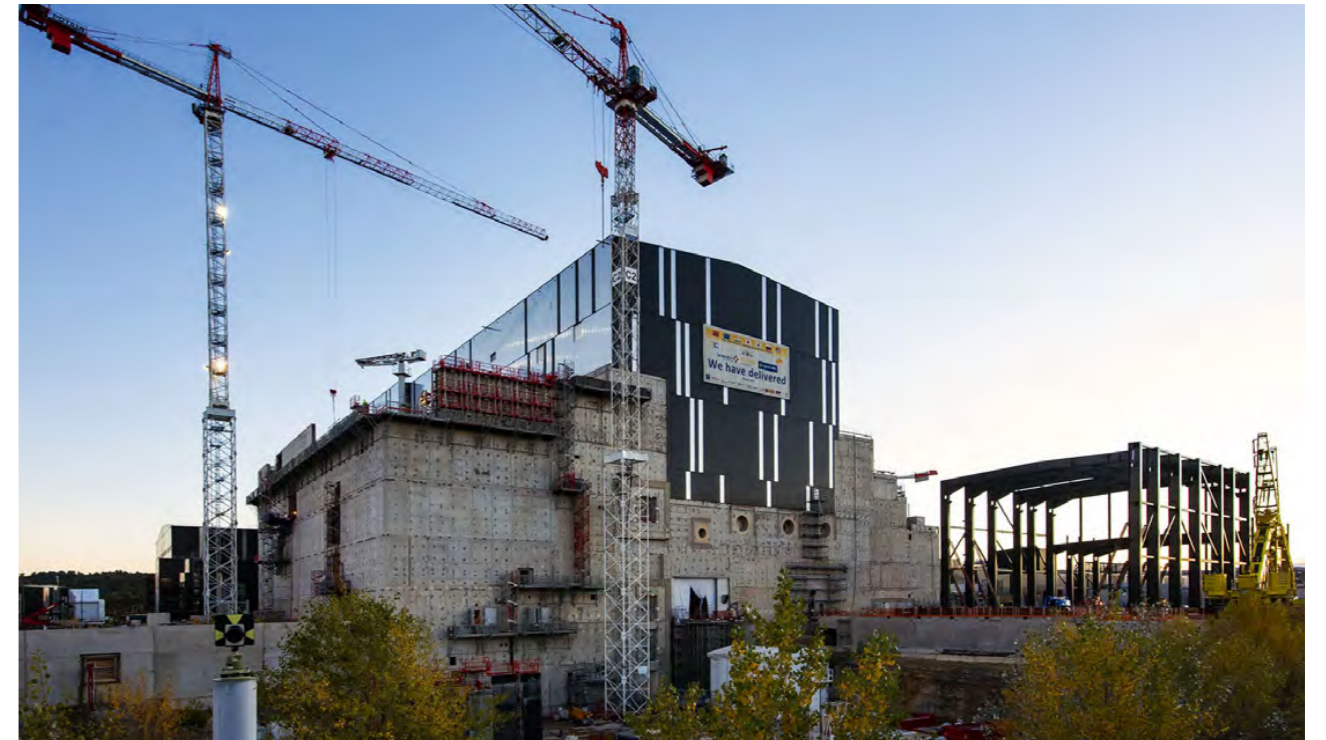
Last level of concrete poured at Level 5, bringing the structure to full length. December 2022 © ITER Organization
