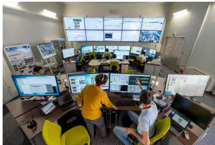
Commissioning and operation from the central control room. Rokkasho. © IFMIF/EVEDA
