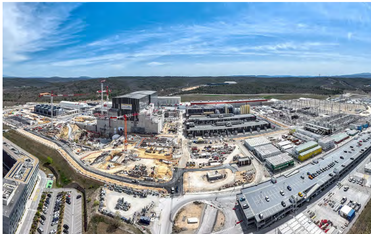
Caption: Aerial view of the ITER site, Cadarache, France © ITER Organization
