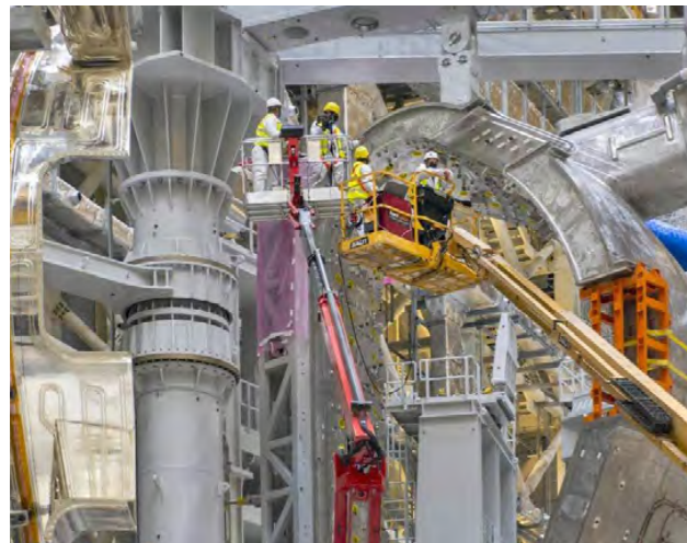
The teams working on the second vacuum vessel sub-assembly. The thermal shield will be rotated toward the vacuum vessel sector and attached in place. January 2022. ©ITER Organization
