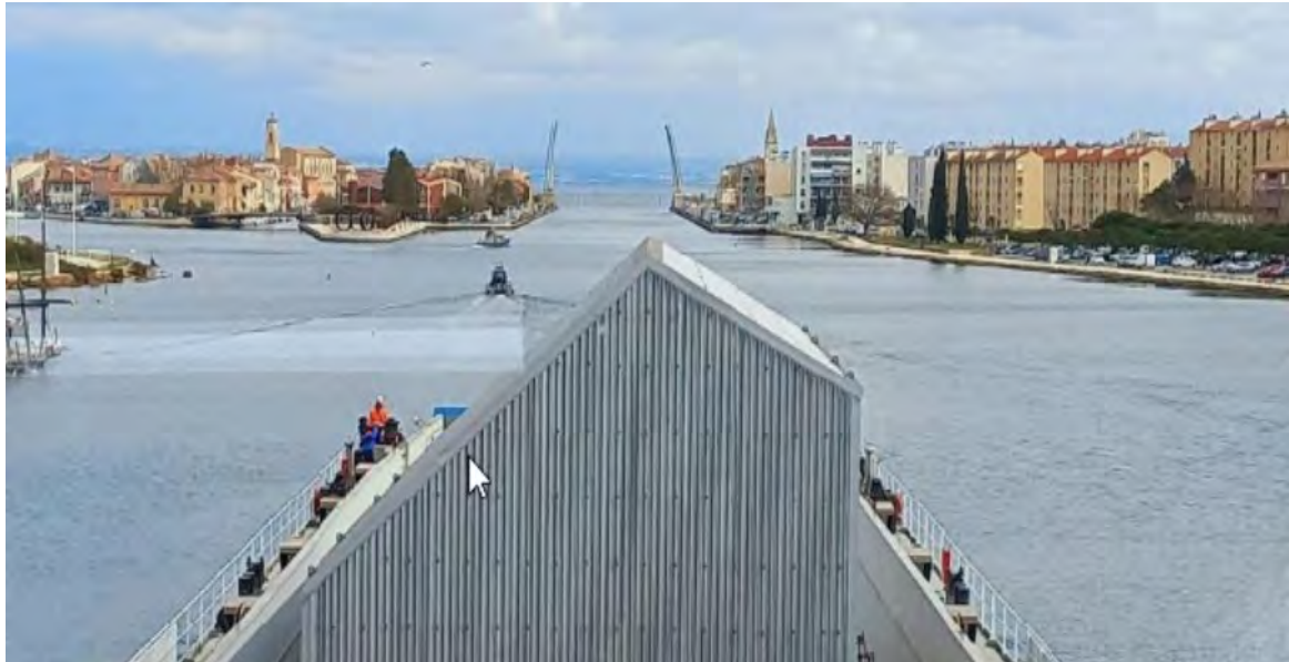
Figure 56: KO-DA VV sector during the Barge transfer from Fos sur mer to La Pointe harbour with the opening of the Martigues Bridge in March 2022 then transported during 4 nights to the ITER Site and arrived the 1st of April 2022. The picture captures the openin
