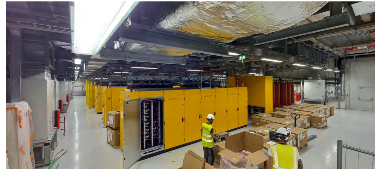
The first of Europe's ECPS were installed in ITER, ready for commissioning. June 2023. ©F4E
