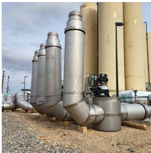
Figure 23: Delivery of quench line header to site (last cryoplant component).
