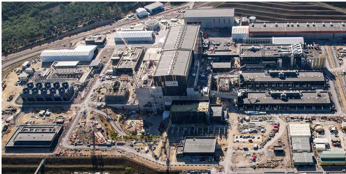
Figure 1: Aerial view of the ITER construction site. Photo: ITER Organization (September 2023)
