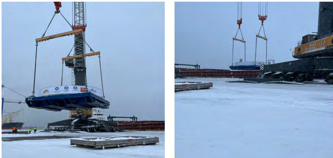
Loading of PF1 into vessel KEIT
