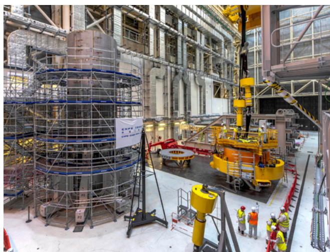
A fourth module was installed on top of the existing central solenoid stack in the ITER Assembly Hall. The US is procuring the six central solenoid modules plus one spare. December 2024. ©ITER Organization
