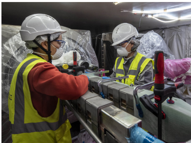
Workers from the CNPE consortium finalised the joints on the feeders procured by China, which will provide electrical power and cooling fluids to the ITER magnets. April 2024. ©ITER Organization
