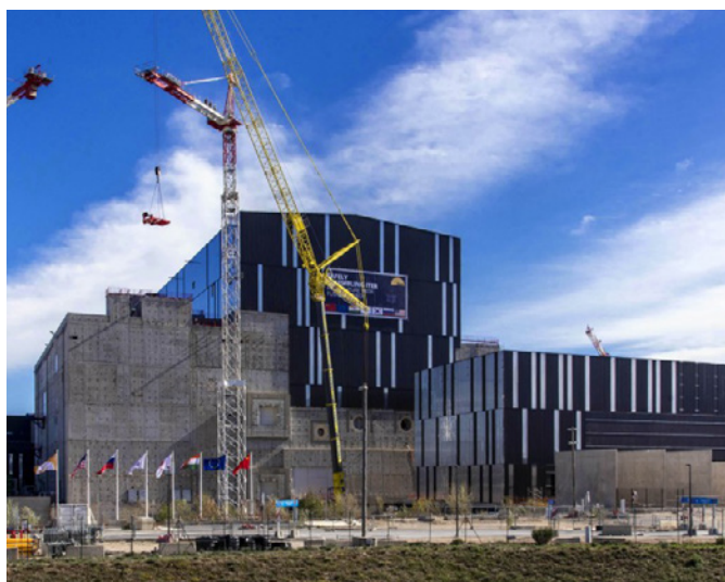
The 84-metre-tall crane next to the Tokamak Complex was dismantled after 10 years of service. ©ITER Organization
