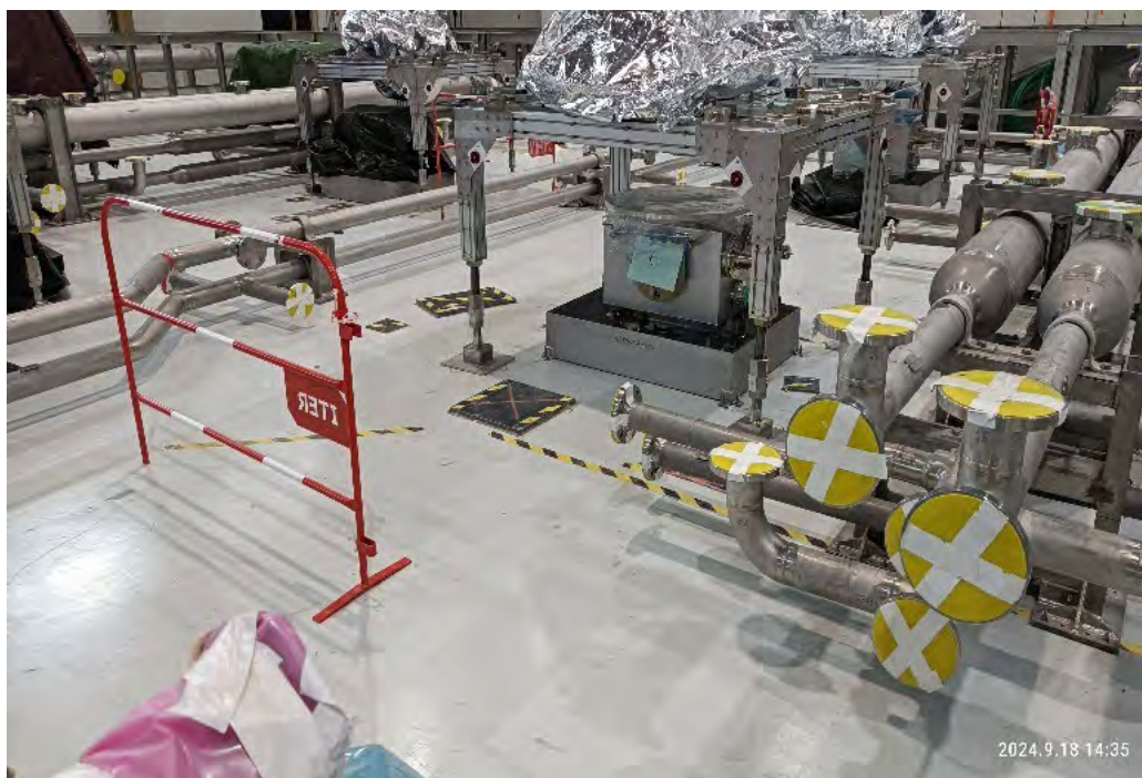
Figure 45: ITER B15, Level 3 status of activities: installation of main water pipes and false floor support checked.
