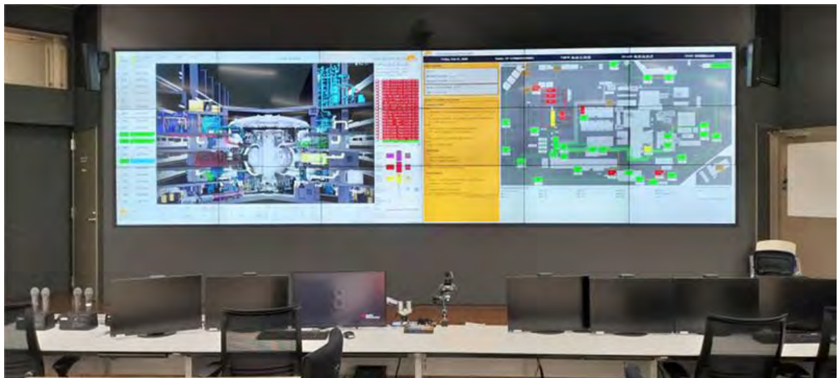
Figure 54: CODAC OPI (OPerator Interface) which is identical to what operators in ITER Main Control Room is watching and (Right) Commissioning Execution Web Page being shown on the REC videowall with 4K resolution
