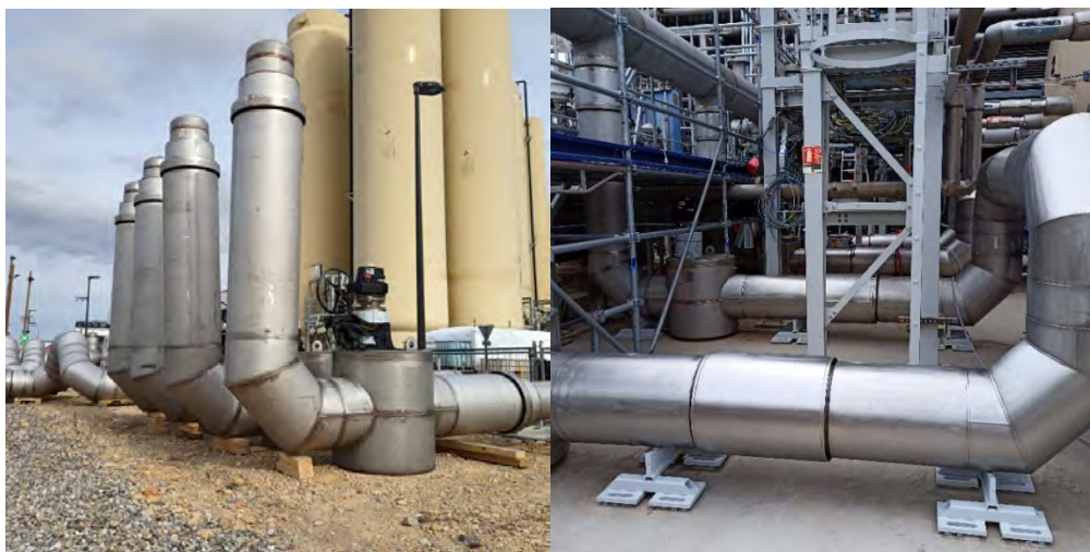
Figure 23: Installed quench line header (last cryoplant component).
