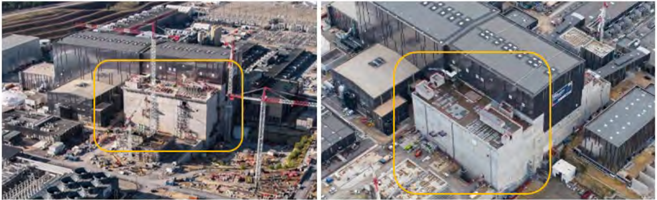
Figure 2: TB18 (Vinci-Ferrovial-Razel, VFR) B14 Tritium Building work status in September 2023 (left) versus October 2024 (right) Photos: © ITER Organization
