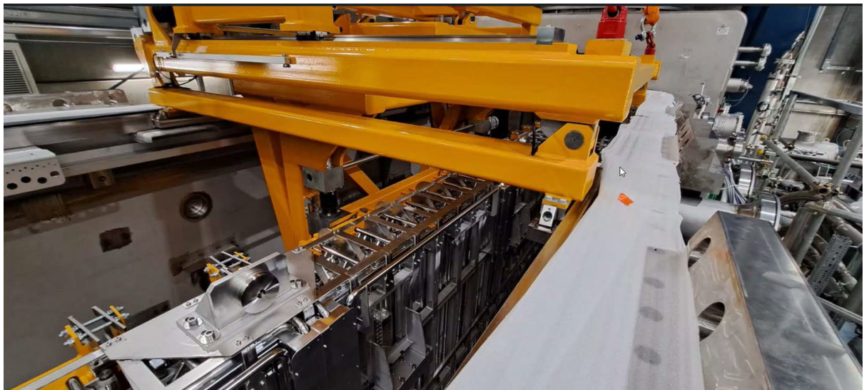
Figure 40: Mitica Cryopump installation detail
