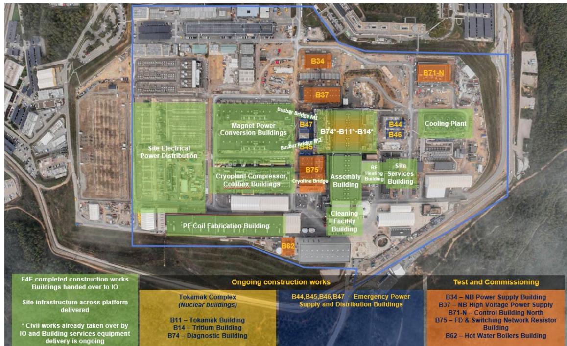
Figure 66: Work site progress end 2024
