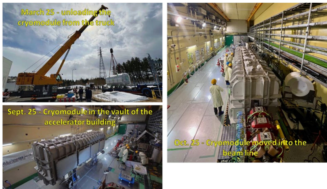
Figure 80: Transfer and integration of the superconducting LINAC into the accelerator beamline
