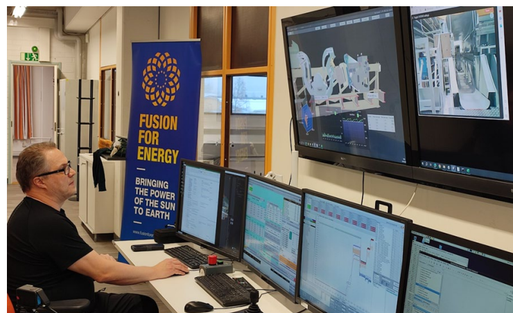
Figure 32: RH Control Room at DTP2
