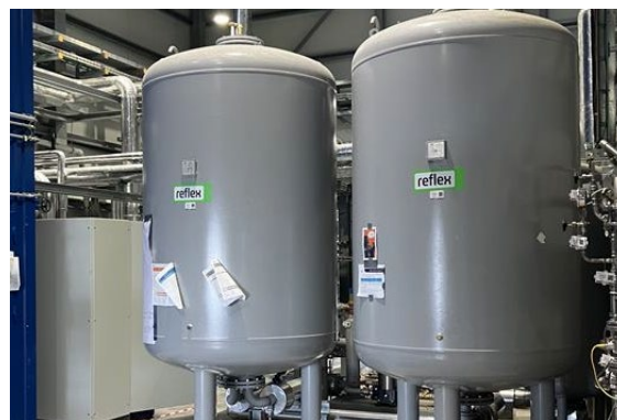
Figure 73: Site Services Building Taken Over by IO
