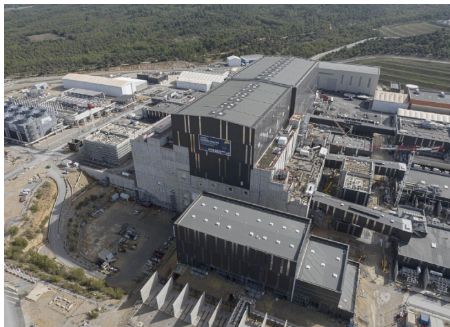
Overview Progress of works
