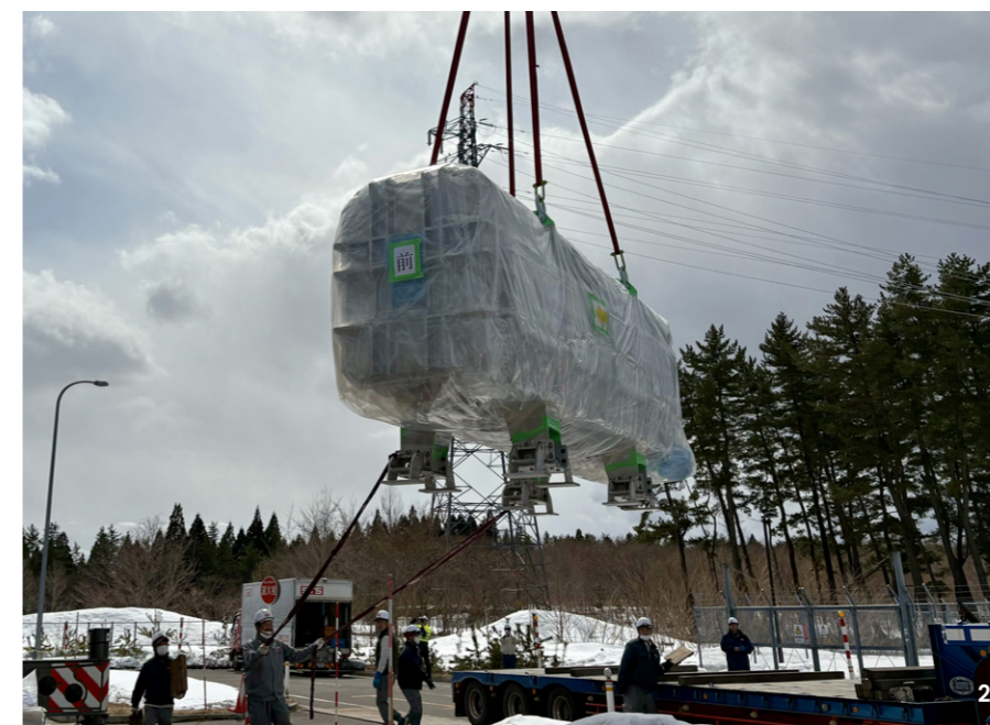
1. Technicians position the SRF linac in the beam line of LIPAc. ©IFMIF/EVEDA 2. Transport of the cryomodule containing the SRF Linac into the accelerator vault in February 2025. ©IFMIF/EVEDA
