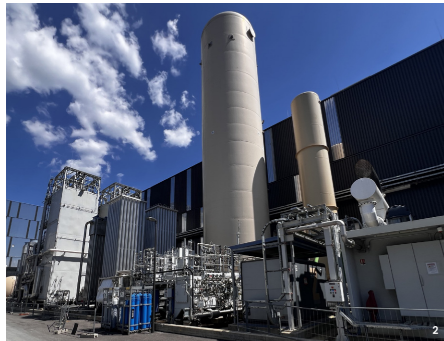
1. The Liquid Nitrogen Plant includes large tanks, compressors and cold boxes. ©F4E 2. Exterior view of the ITER cryoplant, with the liquid nitrogen tank towering over the large facility. April 2025. ©F4E
