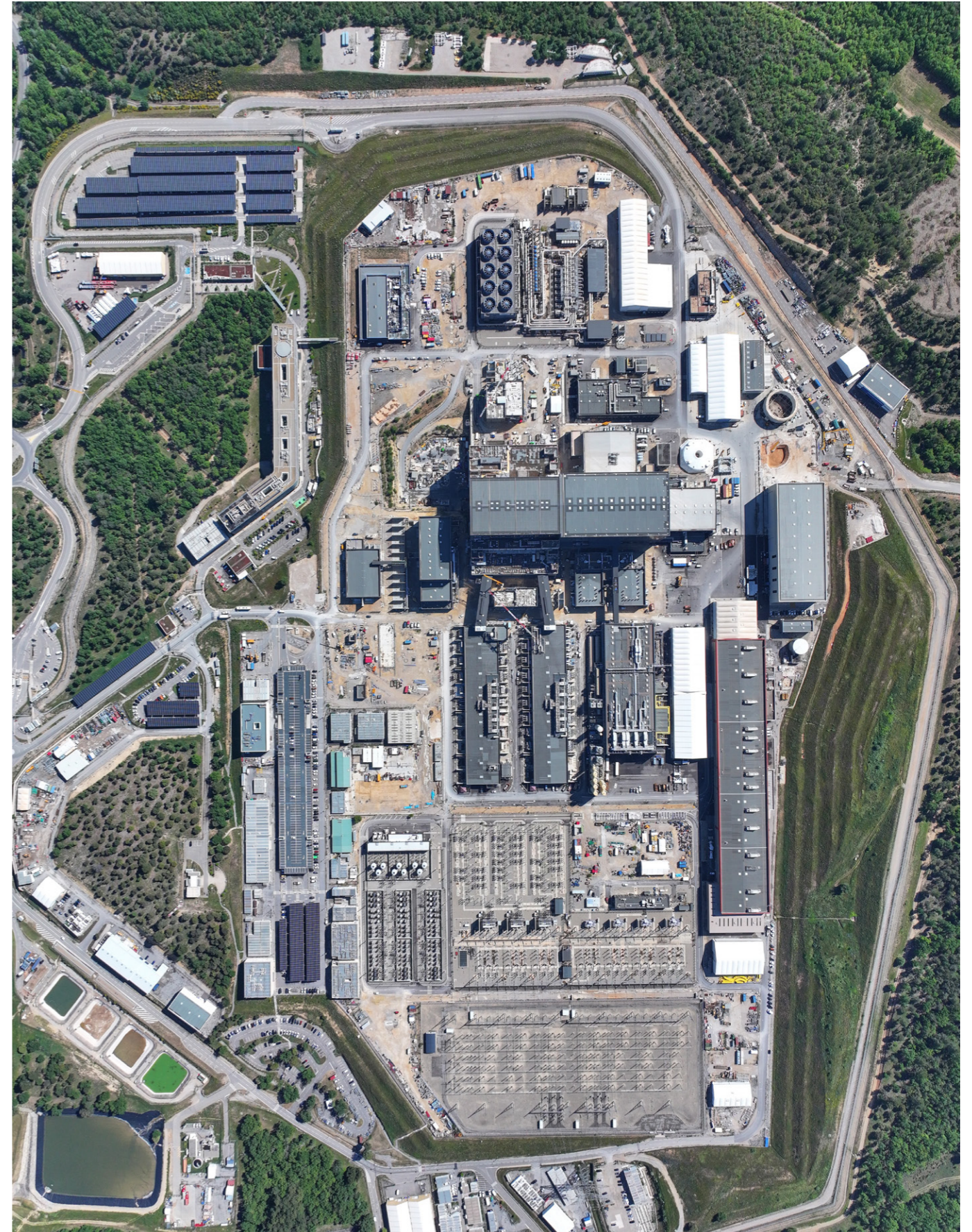
Overhead shot of the ITER site in May 2025. ©ITER Organization / EJV Riche
